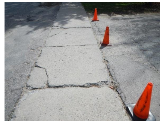
Above: Sidewalks in front of Cutler School have many cracks and are in need of improvements.
