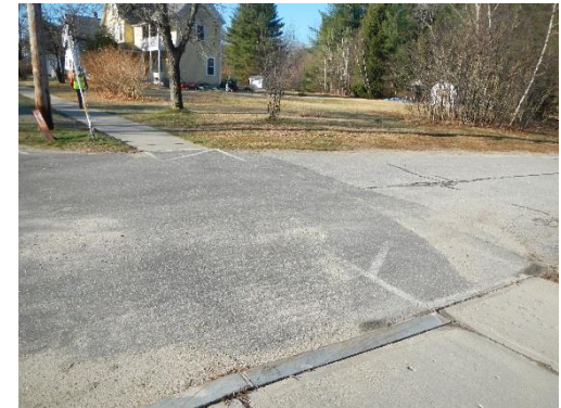
Above: Faded crosswalk in front of the school.
