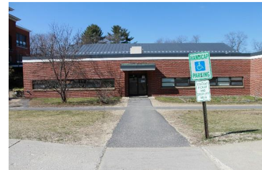
Above: The student drop-off location and school entrance.
