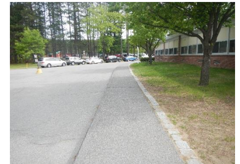
The picture above shows the sidewalk in front of the main entrance to the school and bus drop-off area.
