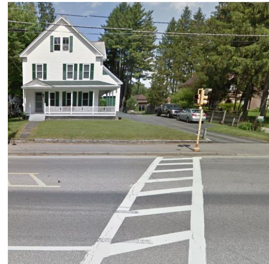
Above: The crosswalk on Park Avenue does not have a curb ramp.
