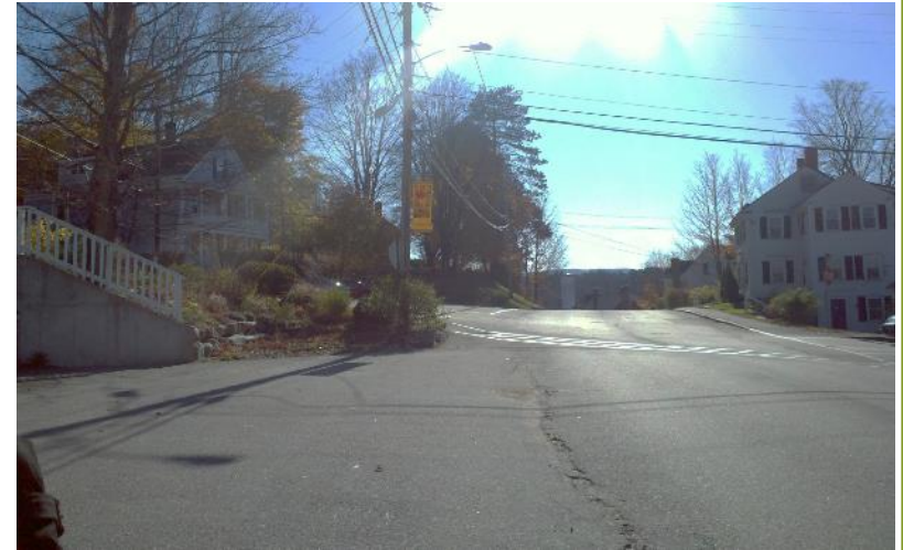
Above photo: This is a view of the intersection from Union Street facing Main Street. The visibility of vehicles or pedestrians entering the intersection from High and Vine Streets is significantly limited.
