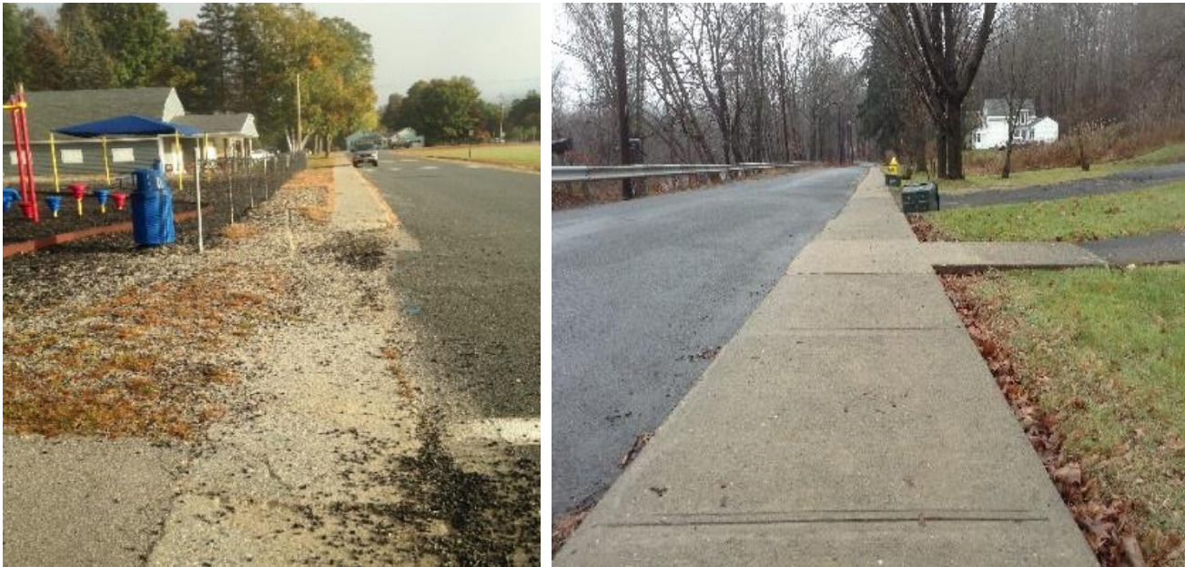
Figure 8 - A section of sidewalk in poor structural condition on School Street (left) and in good structural condition on River Road (right).
