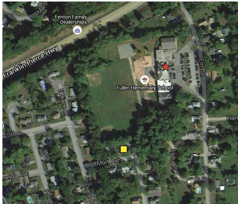
Figures 2 and 3. Aerial views of Fuller Elementary School.
