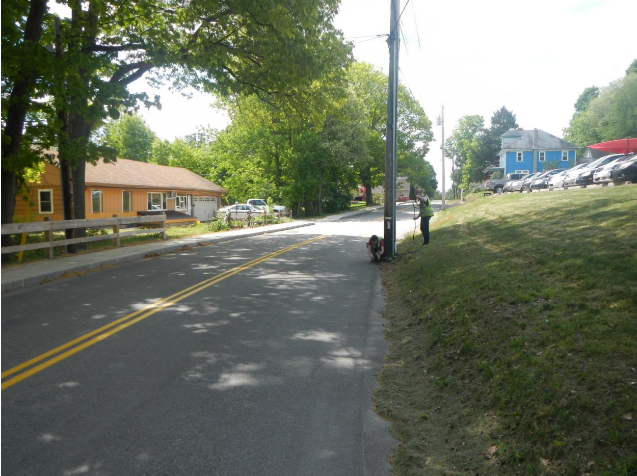
Figure 9 - Site during installation (facing south)
