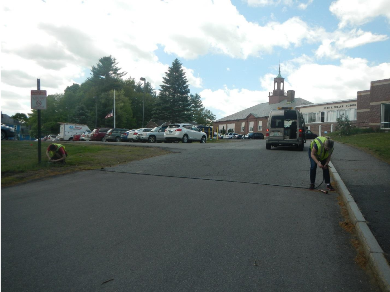
Figure 8 - Site during installation (facing west)
