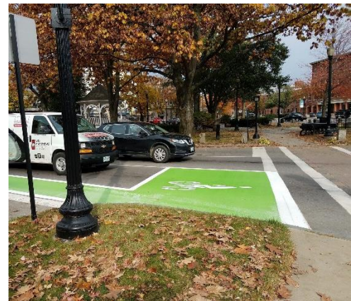
A bicycle box on Central Square in Keene, NH provides space for bicyclists to queue while waiting at a red light.
